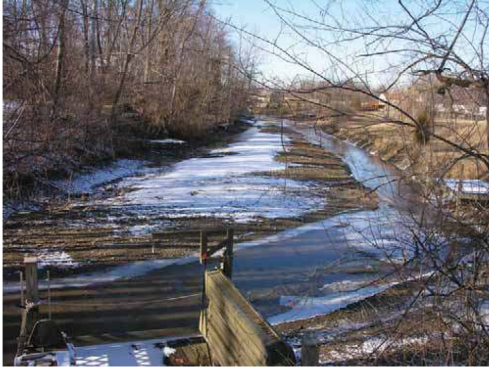
Photograph 1. View from the east end of Straight Creek looking toward the lake. Note the sediment buildup (exposed sand/silt bar) on inside bend (left side) of Straight Creek.
