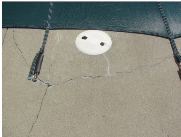
Minor concrete deck cracks
