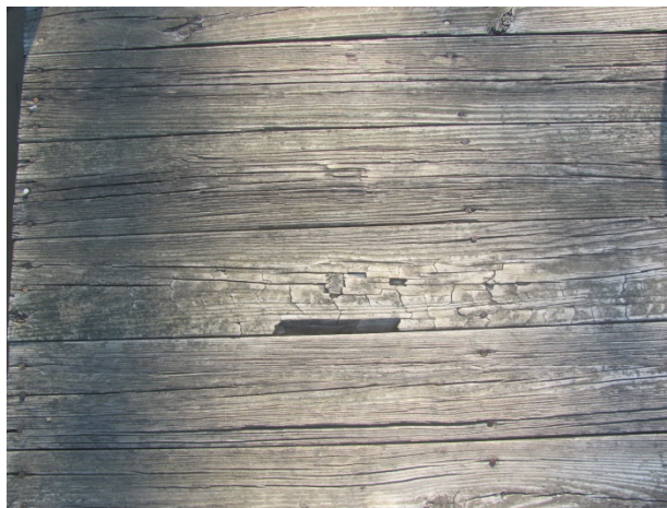
Little Turtle dock, note wood deterioration
