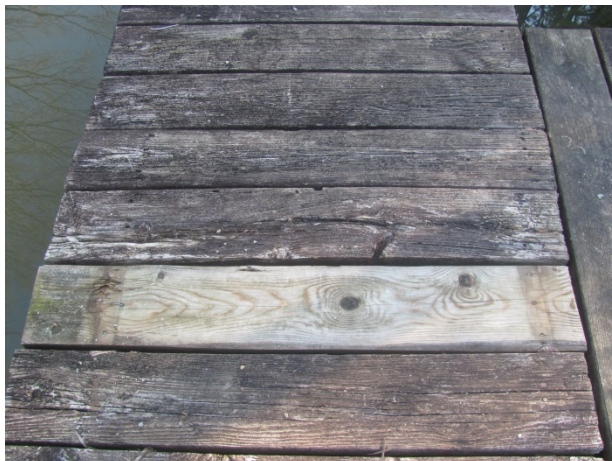
Hiawatha dock, note wood deterioration and previous replacements
