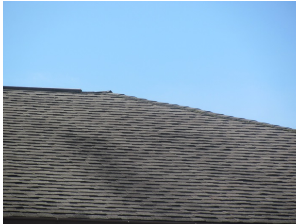
Asphalt shingle roof, note stains
