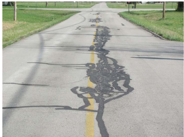
Asphalt pavement at Lake Waynoka Drive, note previous crack repairs
