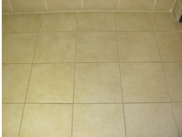
Rest room tile floor coverings, note minor cracks
