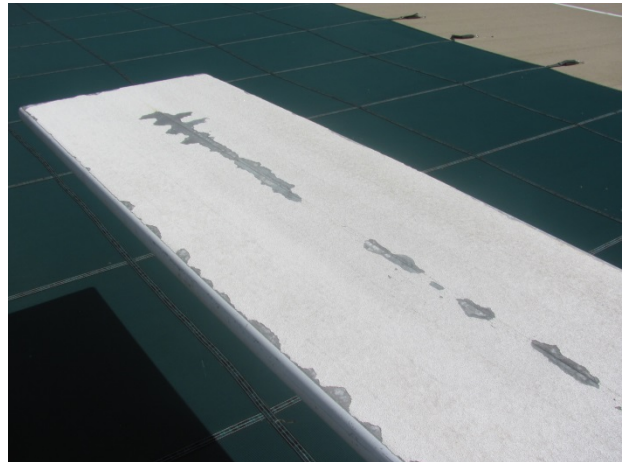
Diving board at main pool, note finish deterioration
