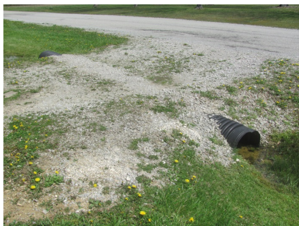
Plastic culvert pipe
