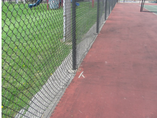
Chain link fence, note isolated warping
