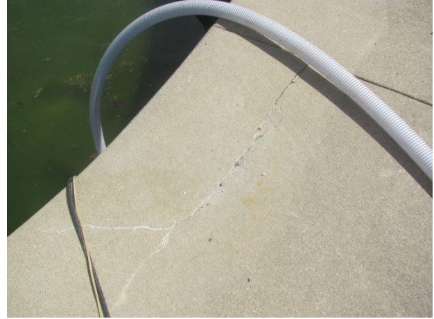
Minor concrete deck cracks
