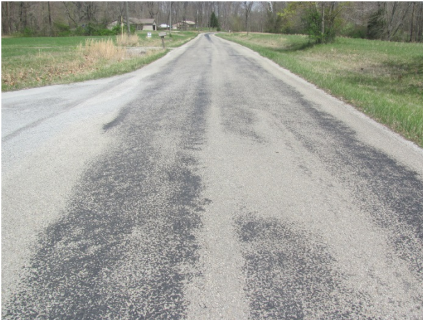
Chip and seal pavement at Sitting Bull Drive, the Association plans to overlay this road with asphalt pavement in 2017
