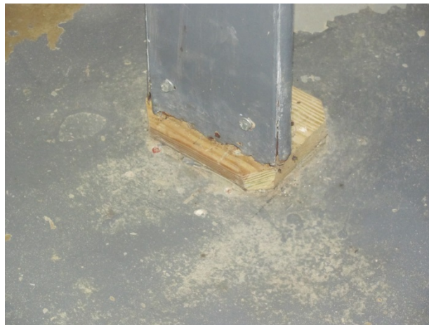
Toilet partition, note rust and previous repairs
