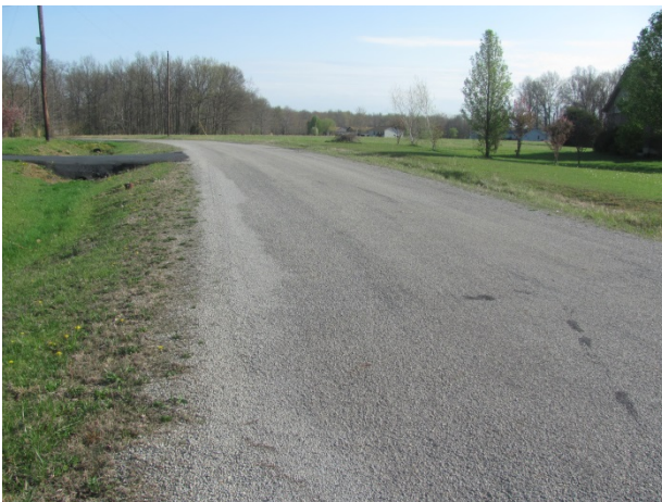
Typical chip and seal road
