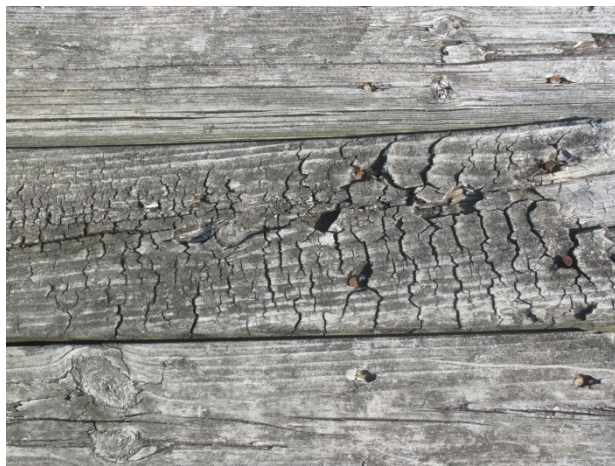
Weathered wood deck board
