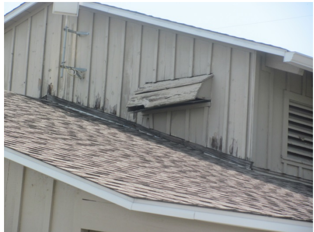
Wood siding deterioration
