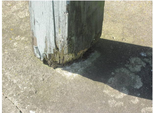
Wood column, note deterioration at base
