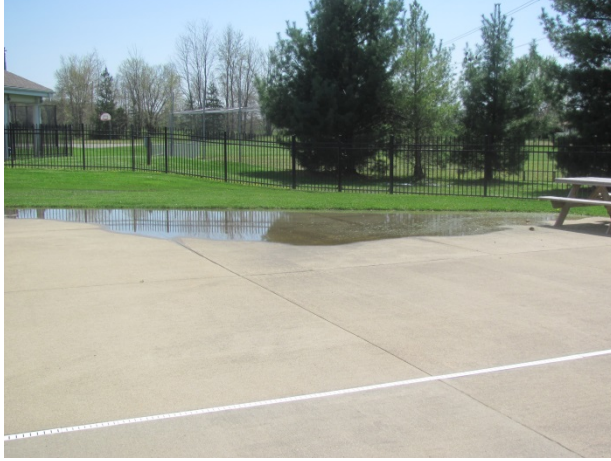
Concrete deck, note standing water
