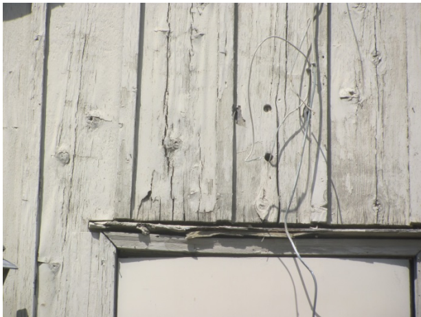
Wood siding deterioration
