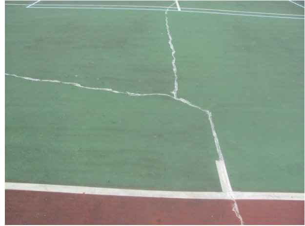
Previous crack repairs
