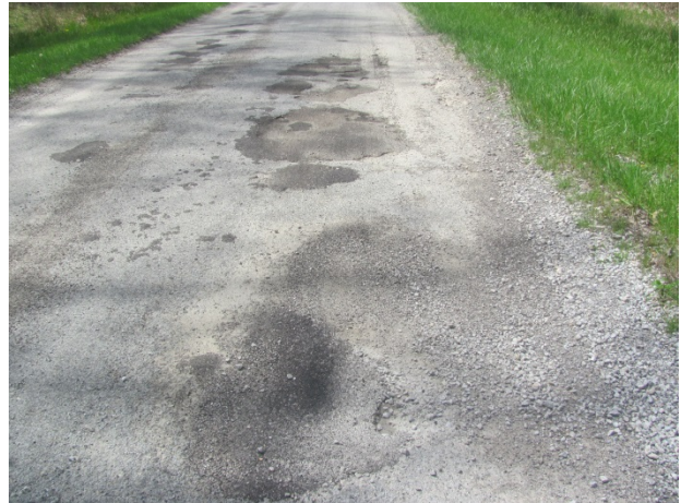
Chip and seal pavement at Yuma Drive, note loose gravel and previous pot hole repairs. The Association plans to overlay this road with asphalt pavement in 2017.
