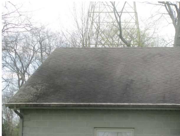
Asphalt shingle roof, note stains and shingle deterioration
