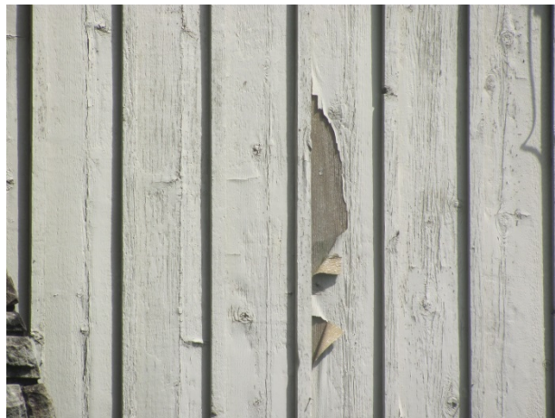
Wood siding deterioration
