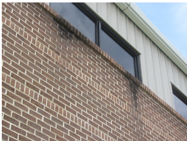
Brick masonry and metal siding, note stains
