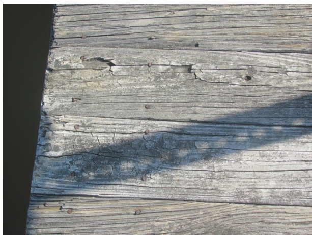
Wood deterioration and rusted nail fasteners
