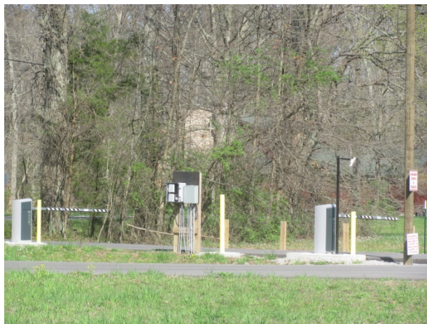
Rear swing arm gates and operators
