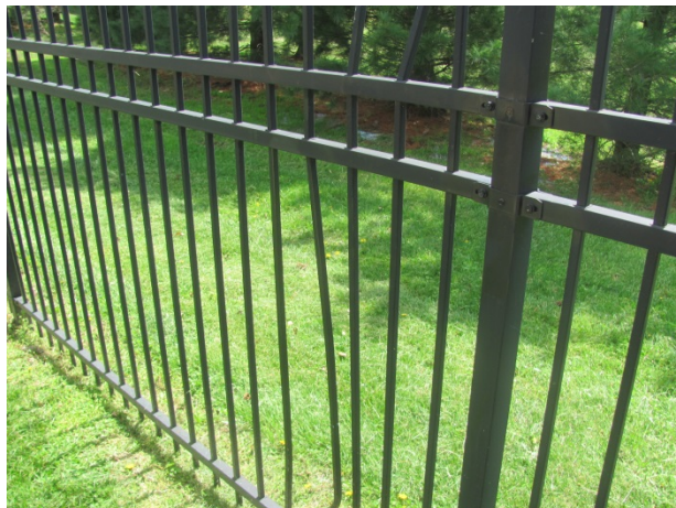
Damaged fence picket
