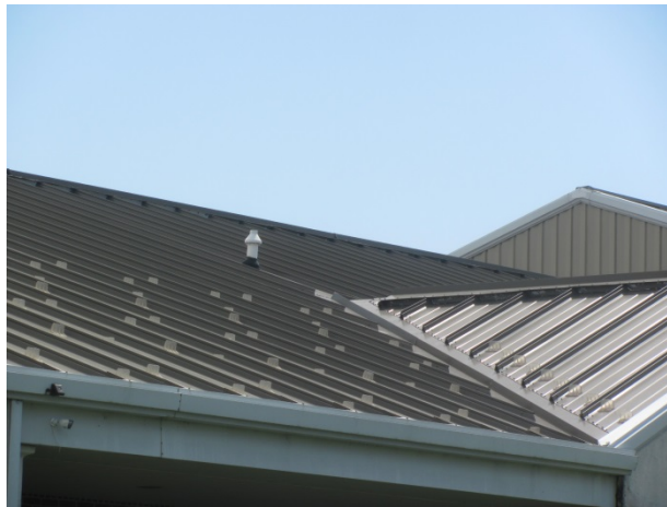
Standing seam metal roof
