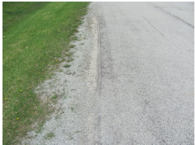
Chip and seal road, note edge deterioration
