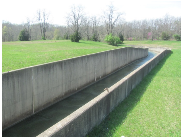
Concrete spillway
