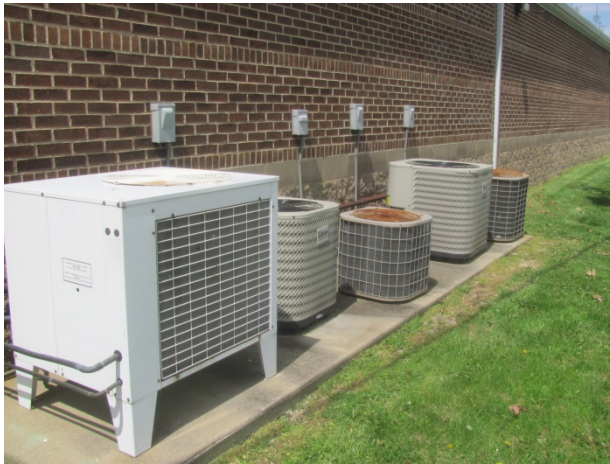
Small condensing units
