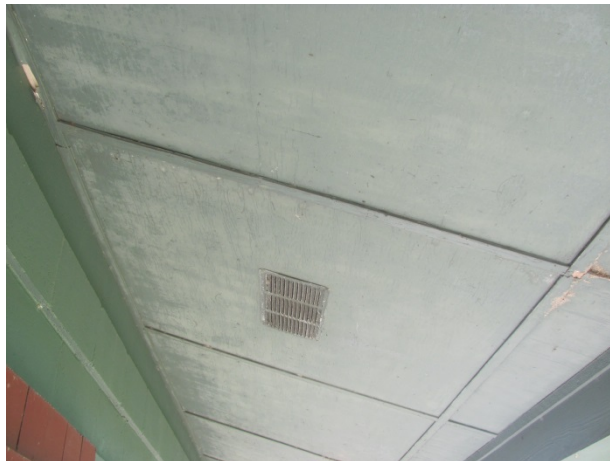
Wood soffits, note faded finishes and wood deterioration
