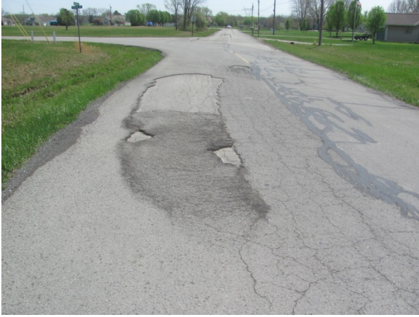
Asphalt pavement at Lake Waynoka Drive, note isolated deterioration near Yuma Drive
