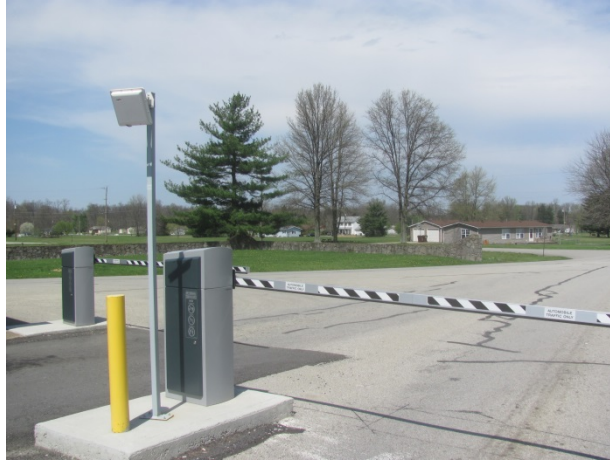
RFID reader and swing arm gate
