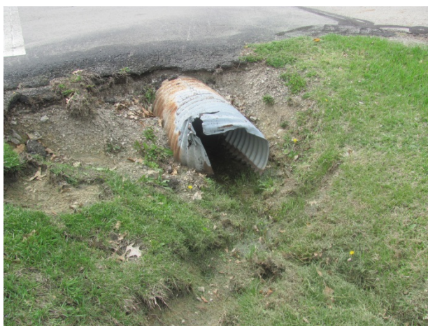
Metal culvert pipe, note rusted and crushed sections
